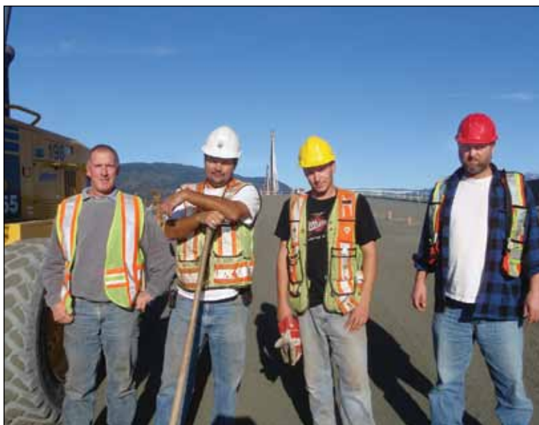
Local 115 members working for B&B Contracting on the south side of the Coast Meridian Overpass.
