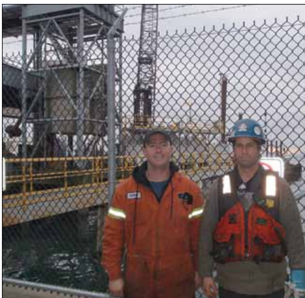
Brothers Travis Cummings and Wes Bauder working for Vancouver Pile Driving at Tsawwassen Ferry Terminal’s Berth 4.
