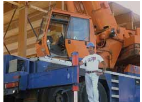
Brother Steve Bird working for Mega Cranes on the new Pitt River Community School.
