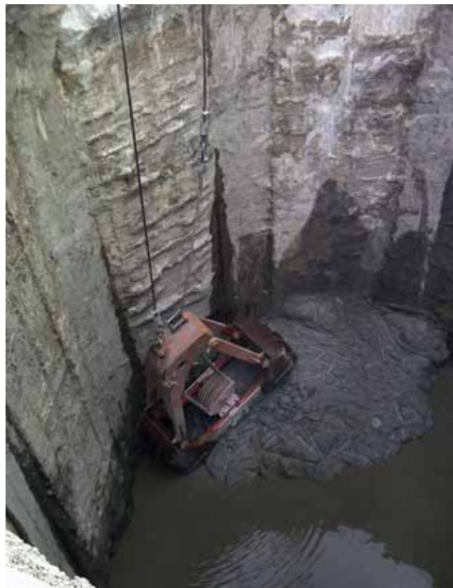
Brother Chris Good operating a crane with a clamshell bucket for McNally-Aecon JV. He's digging out a concrete blockage from a panel pour.
