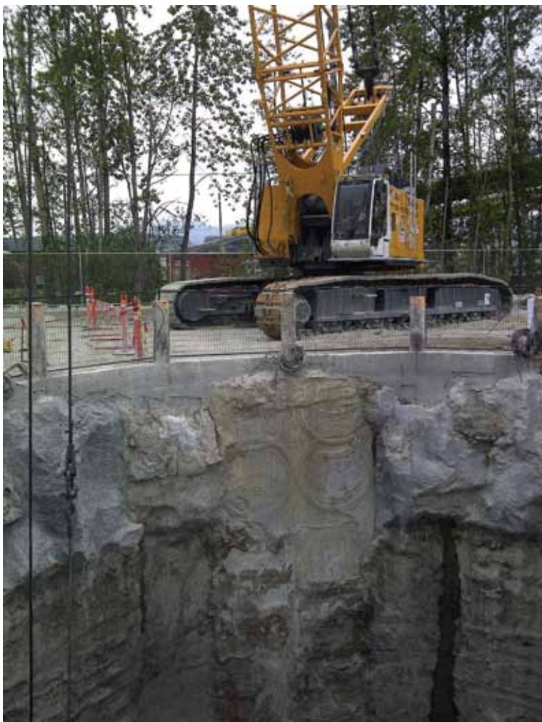
Brother Chris Good operating a crane with a clamshell bucket for McNally-Aecon JV. He's digging out a concrete blockage from a panel pour.
